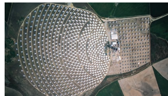
Thermoelectric Solar Platform, Sevilla, Spain © Abengoa
